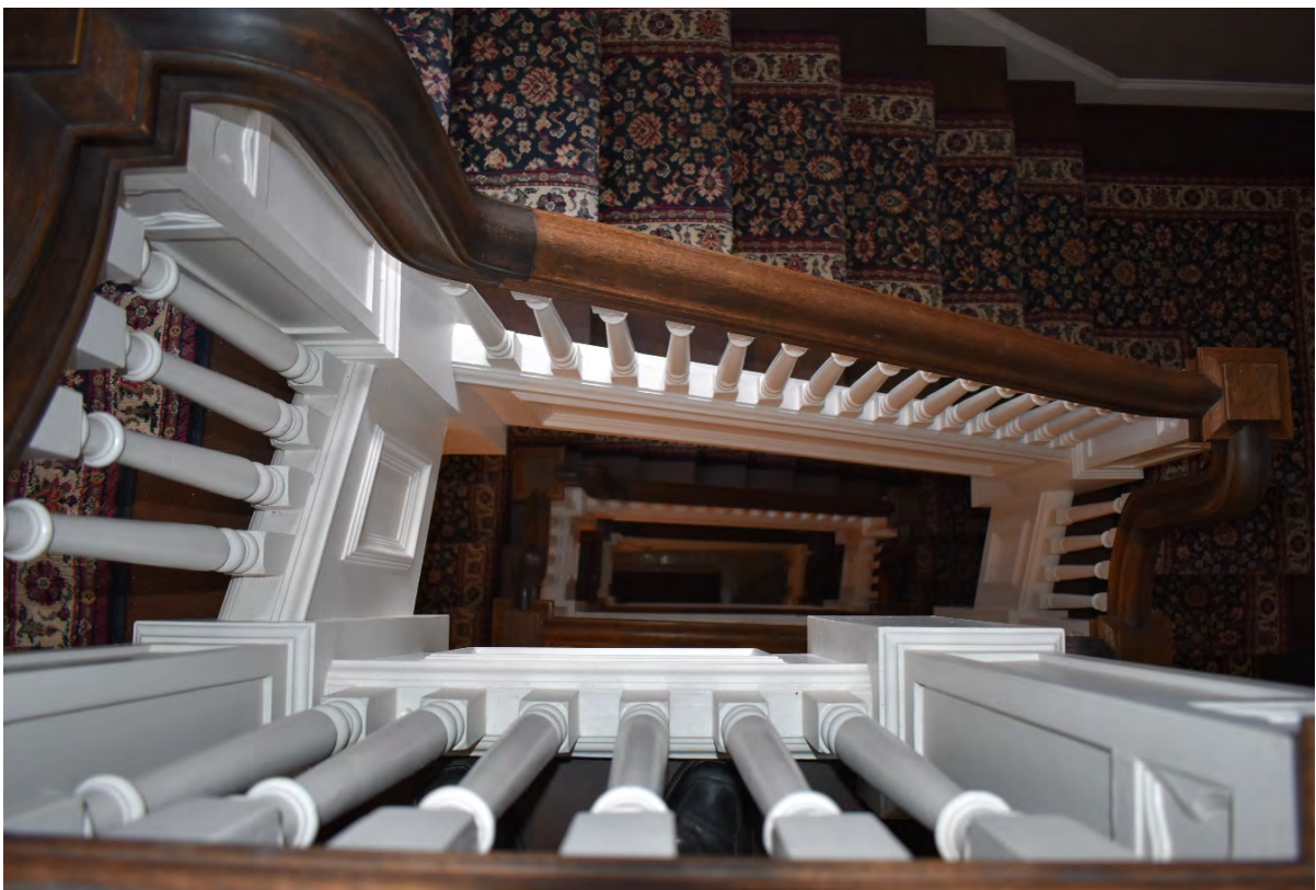
Fig. 59 – Interior, south entry stairwell.
