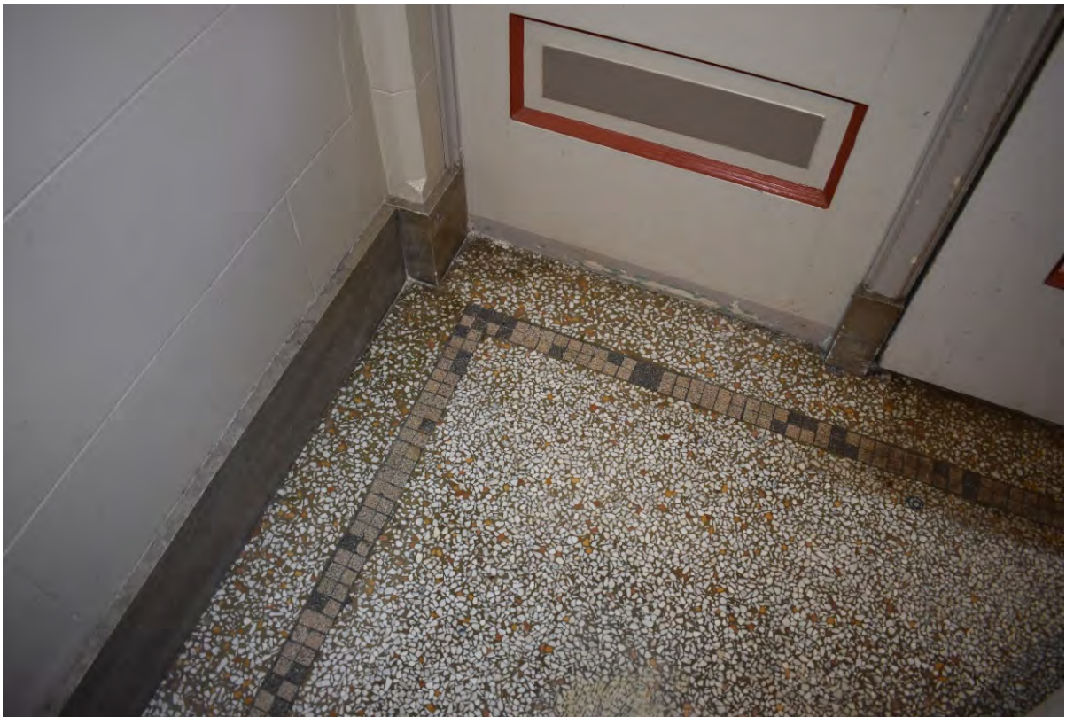
Fig. 37 – Interior, east entry vestibule, showing terrazzo flooring.
