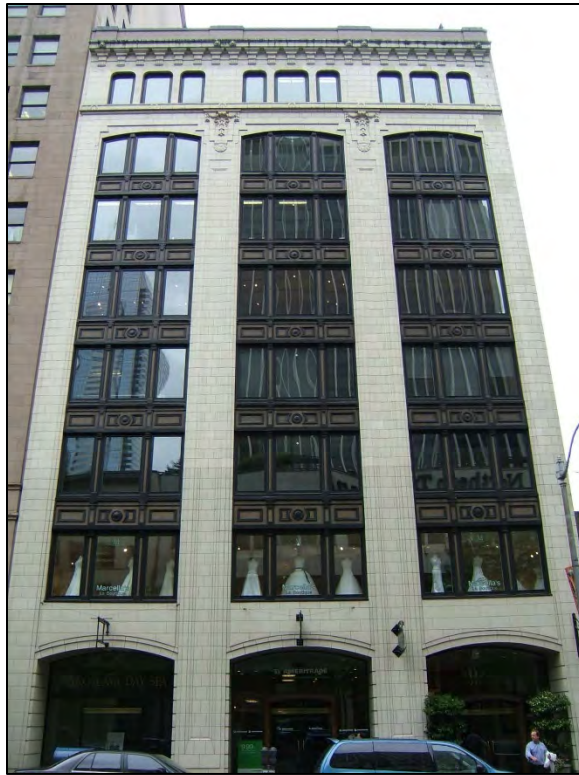
Fig. 78 – Holland Building (1920; upper four floors by Stuart & Wheatley, 1923) (DON)
