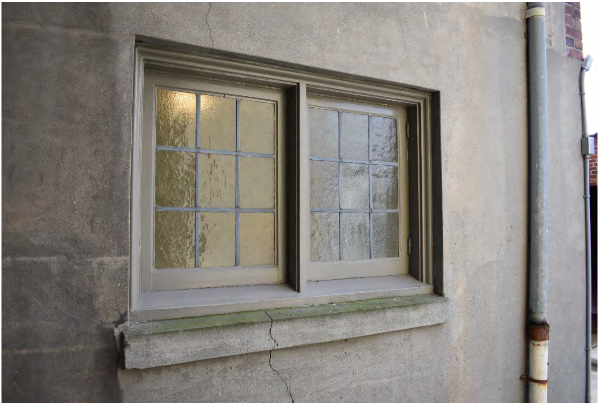
Fig. 30 – West elevation, lightwell courtyard, showing an original leaded glass window.
