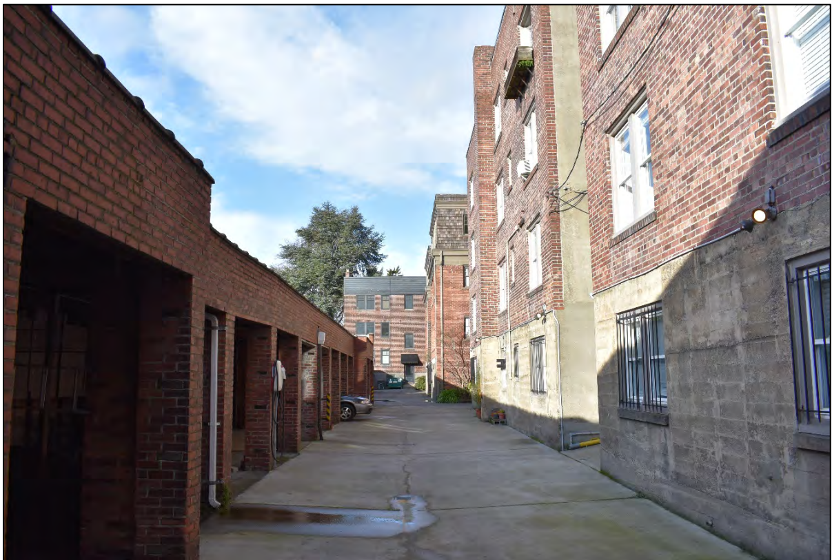
Fig. 19 – West elevation at right; garage at left. Two adjacent apartment buildings visible in distance.
