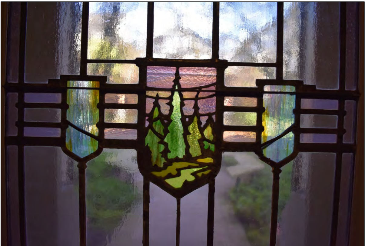
Fig. 35 – Interior, east entry vestibule, detail front door.
