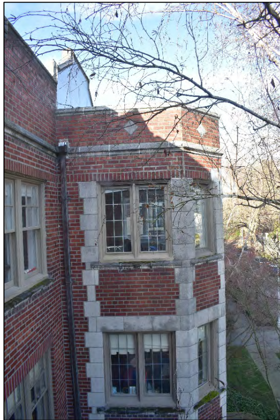
Fig. 63 – Interior, upper floor at south end, typical unit, view from sunroom.
