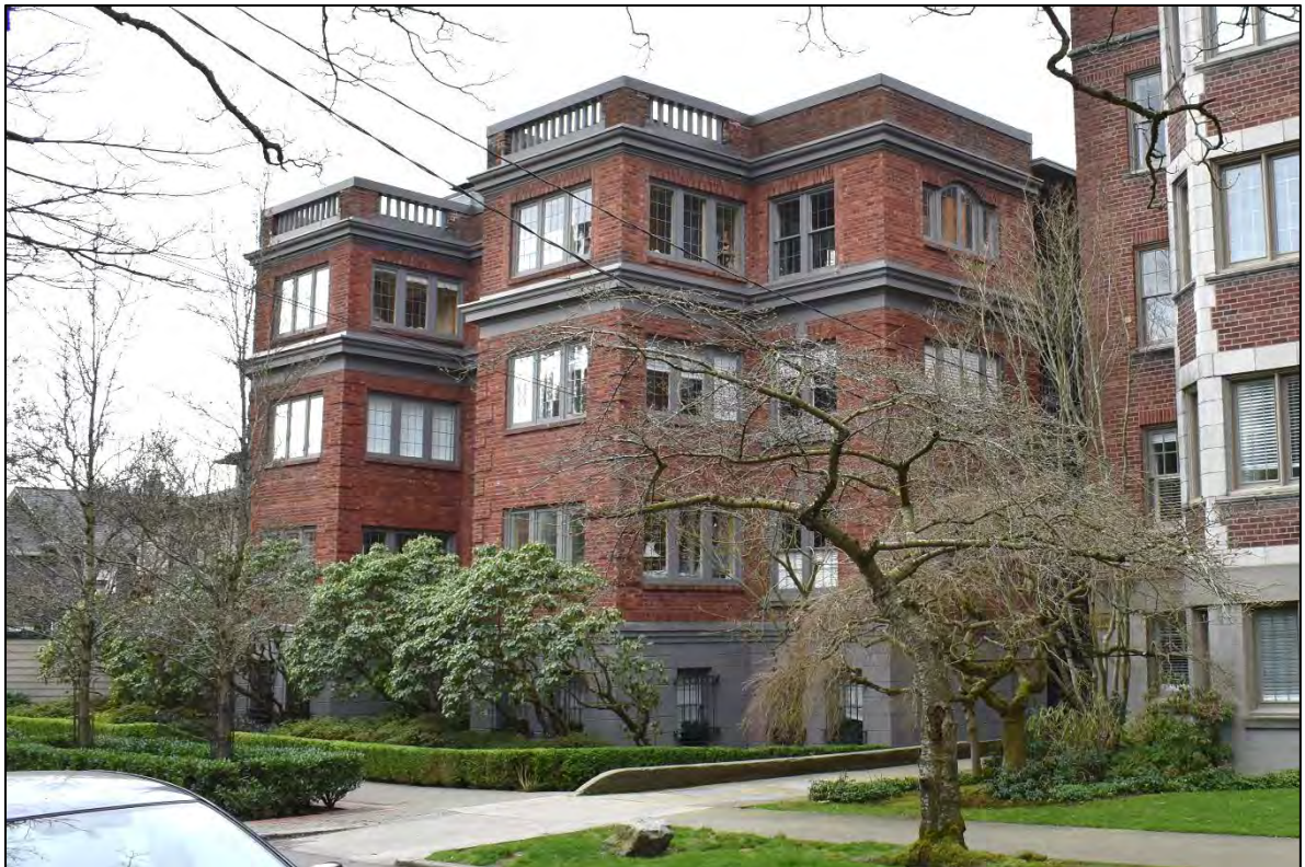
Fig. 9 – Context: The Parkview Apartments (George W. Stoddard, 1922) at 921 11 th Avenue E., next door to the subject property.
