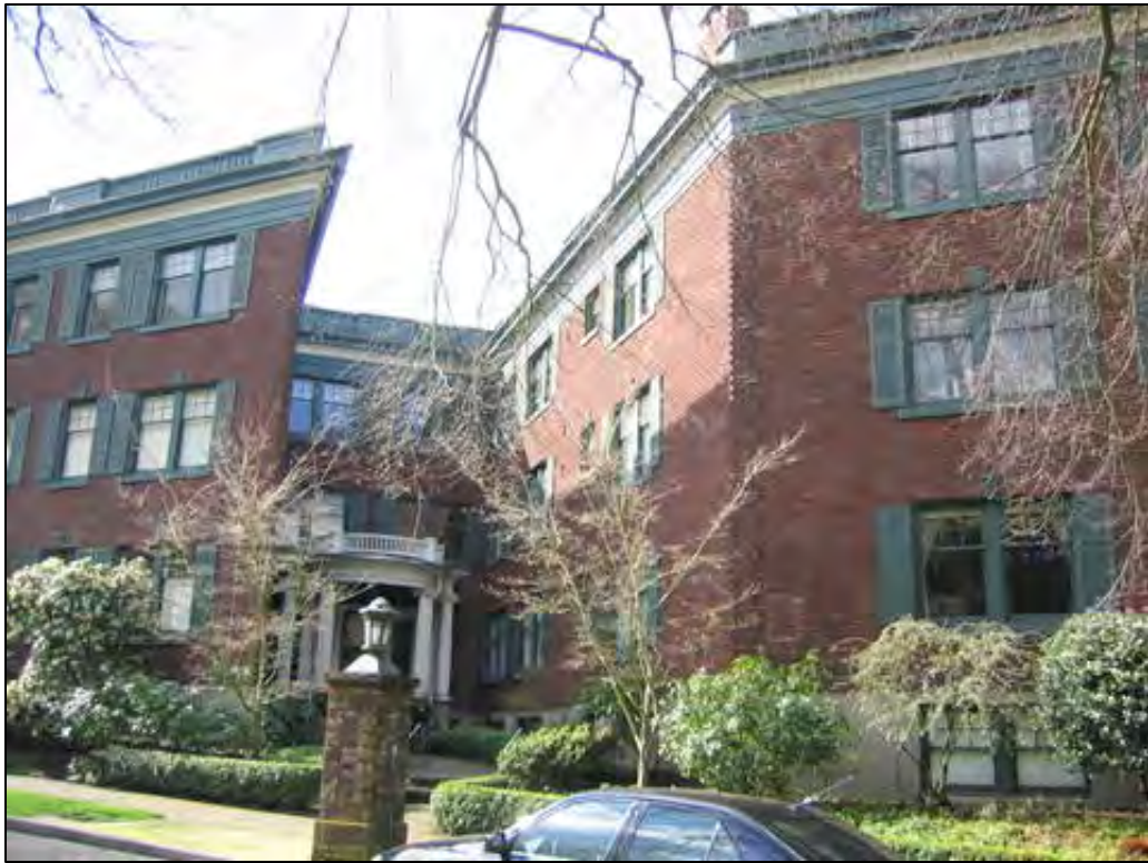
Fig. 10 – Context: The Washington Arms Apartments (Victor Voorhees, 1919) at 11 th & Prospect. (DON)
