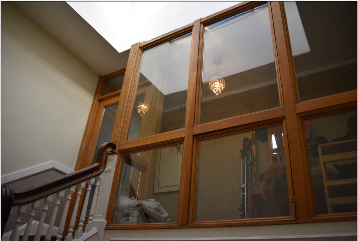
Fig. 57 – Interior, upper floor at north end, upper part of main entry stair, showing glazed wall at top of stair which creates a double penthouse unit. Skylight also visible upper left.
