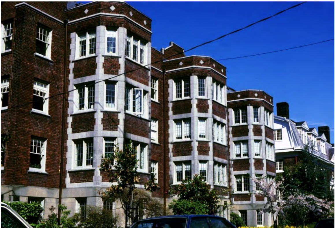
Fig. 77 – 1975 photo of the subject building, detail of bays. (SMA 182134)
