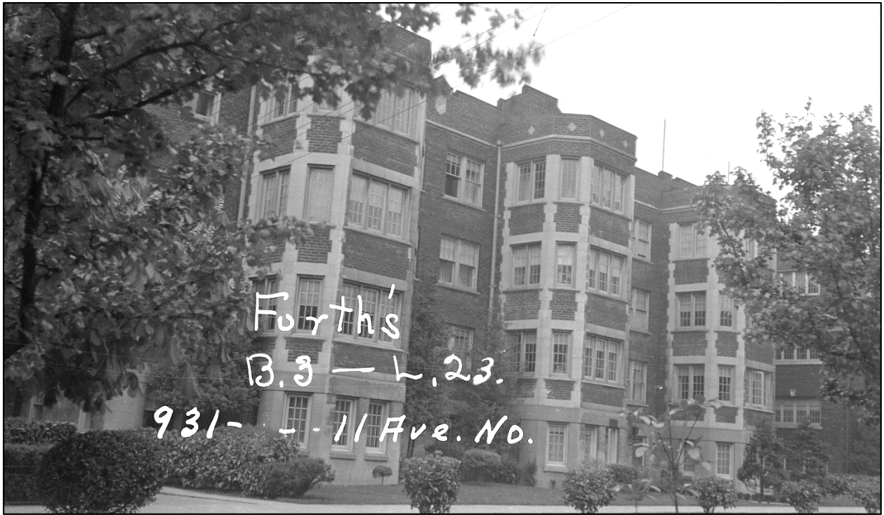
Fig. 72 – 1937 Tax Assessor photo of the subject building.
