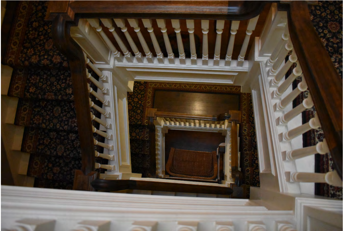
Fig. 56 – Interior, upper floor at north end, upper part of main entry stair.
