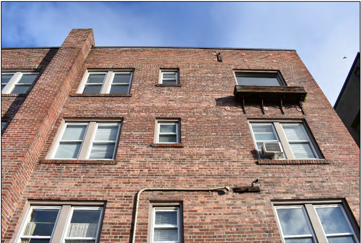
Fig. 23 – West elevation, north part of building, upper floors, south half.
