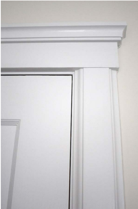
Fig. 54 – Interior, upper floor at north end, typical unit, showing door trim.
