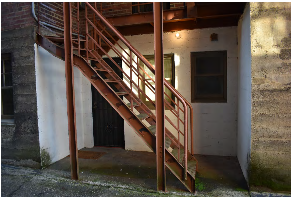
Fig. 33 – North elevation, fire exit stair.
