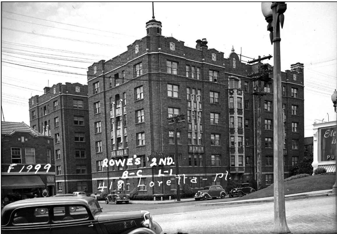
Fig. 79 – Biltmore Apartments (1923) (King County Tax Assessor)
