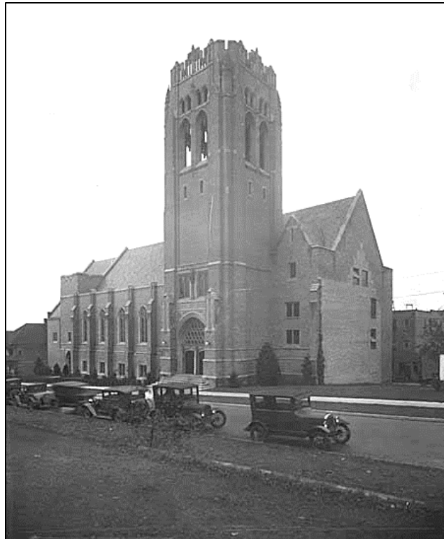
Fig. 91 – Sylliaasen & Sando, builders: University Temple United Methodist Church (1927) (MOHAI WSColl 1983.10.3566)
