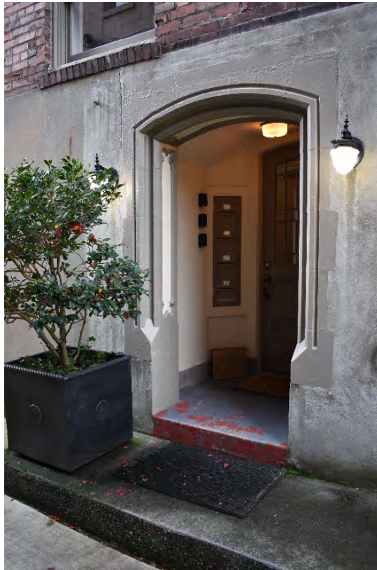
Fig. 18 – South elevation, detail of side entry serving southern third of building.
