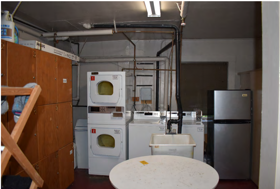
Fig. 41 – Interior, first floor, laundry room.
