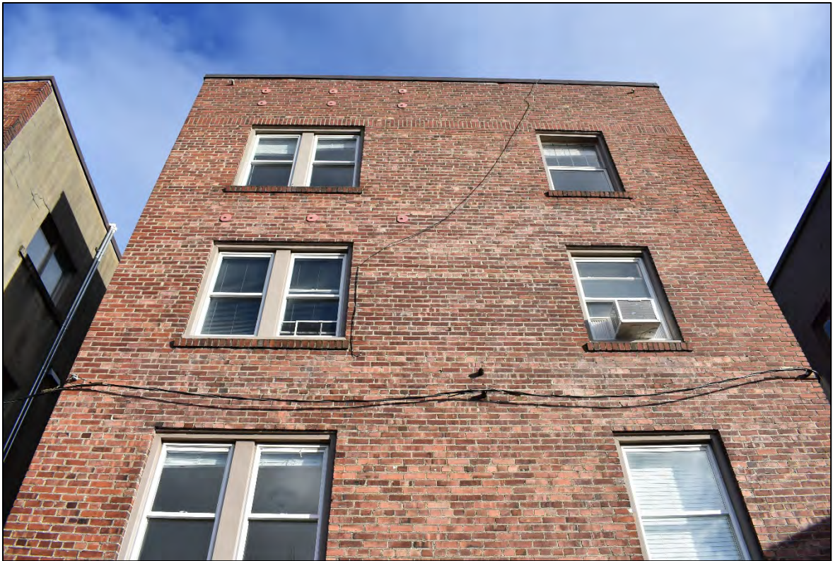
Fig. 24 – West elevation, south part of building, upper floors.
